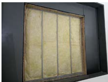
1 #1050R Self-Adhesive Tape, applied to the studs
