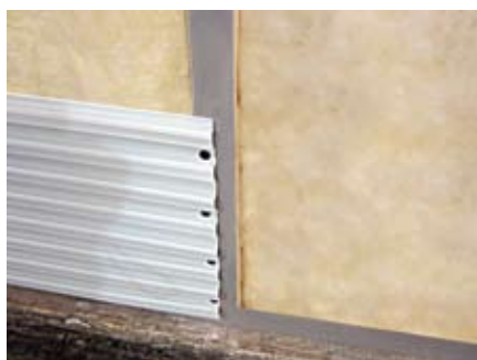
2 #1033 - Primary Insulator, fastened horizontally to the studs
